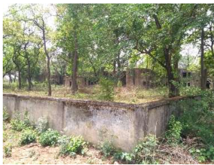
Abandoned health care centre
