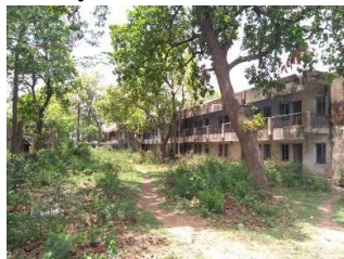
Abandoned Industrial Training Institute
