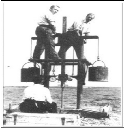
Figure: 2. 31 Early CPT rig in between 1930 to 1940 (Robertson and Cabal 2015)
