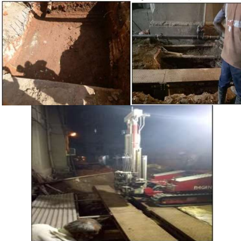
Figure: 4.3 Photographs of test pit and test set up
