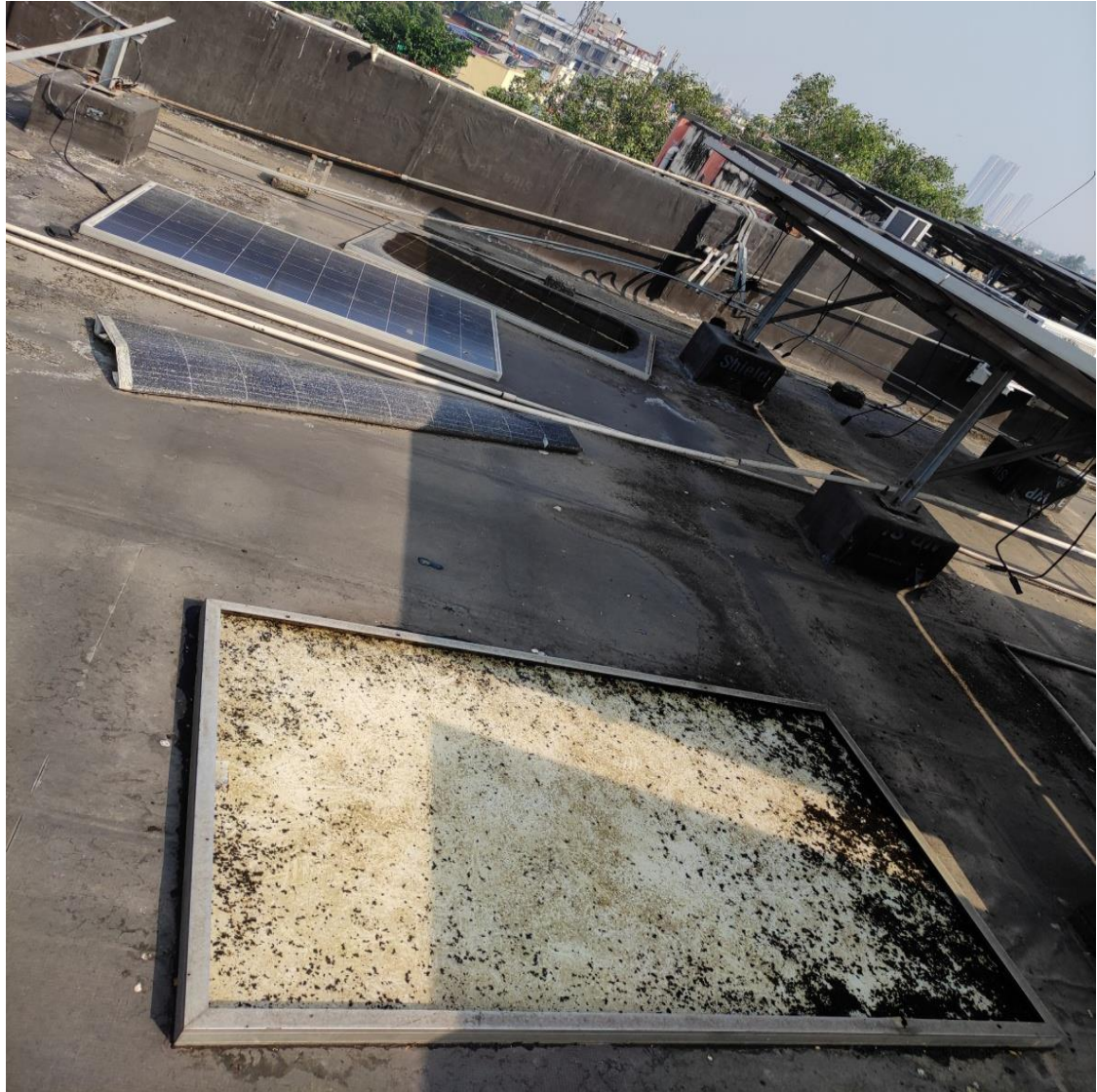
Fig. 3.1: Damaged areas of the Solar Plant.
