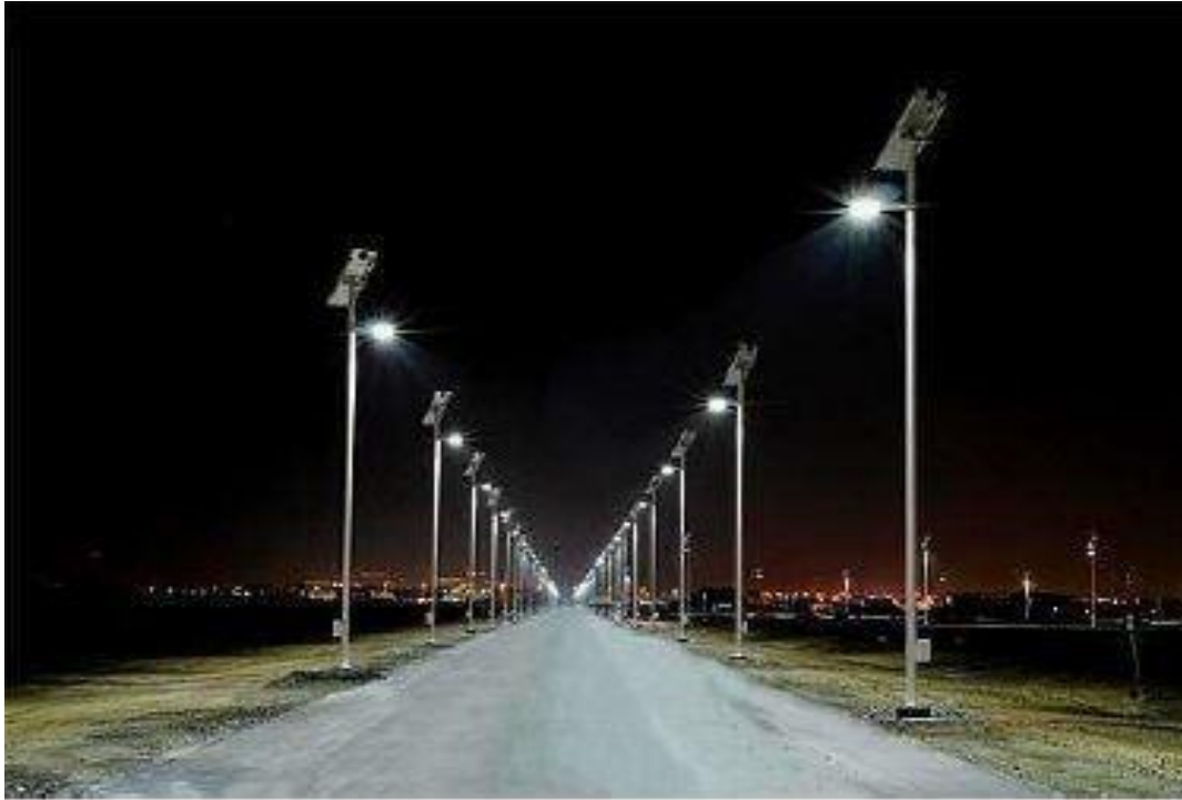
Fig.3.2: Solar LED luminaire with SPV panel
