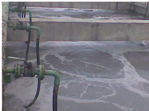
Fig. 3.4 Aeration tank for biological treatment unit at CETP, Bantala
