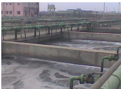
Fig. 3.4 Aeration tank for biological treatment unit at CETP, Bantala
