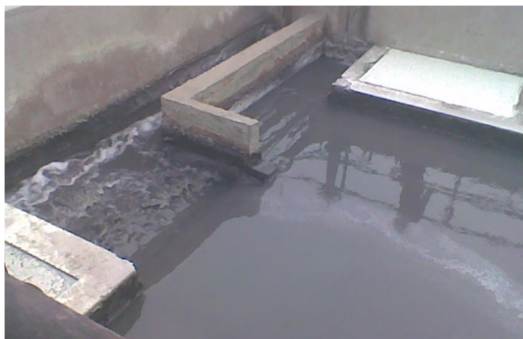
Fig. 3.2 Settling tank for raw composite effluent
