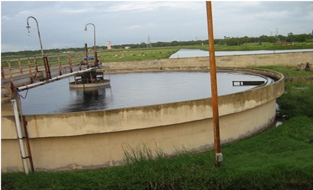
Fig. 3.1 A typical secondary clarifier in CETP plant
