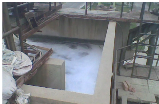
Fig. 3.3 Primary clarifier for raw composite effluent
