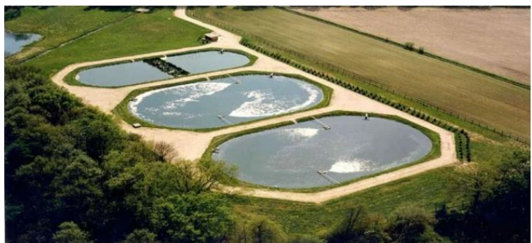
Figure 6. 18 : Aerated Lagoon System
