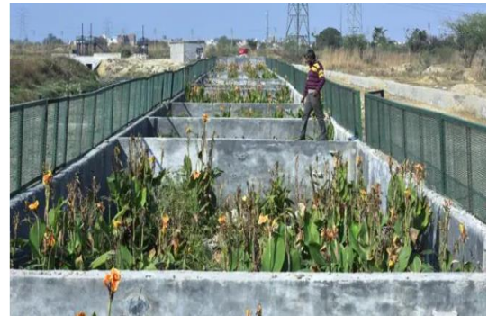
Figure 9. 4 : A view of a pilot Sewage Treatment Plant (STP) that is built with pebbles and plants, at Bawana, in New Delhi
