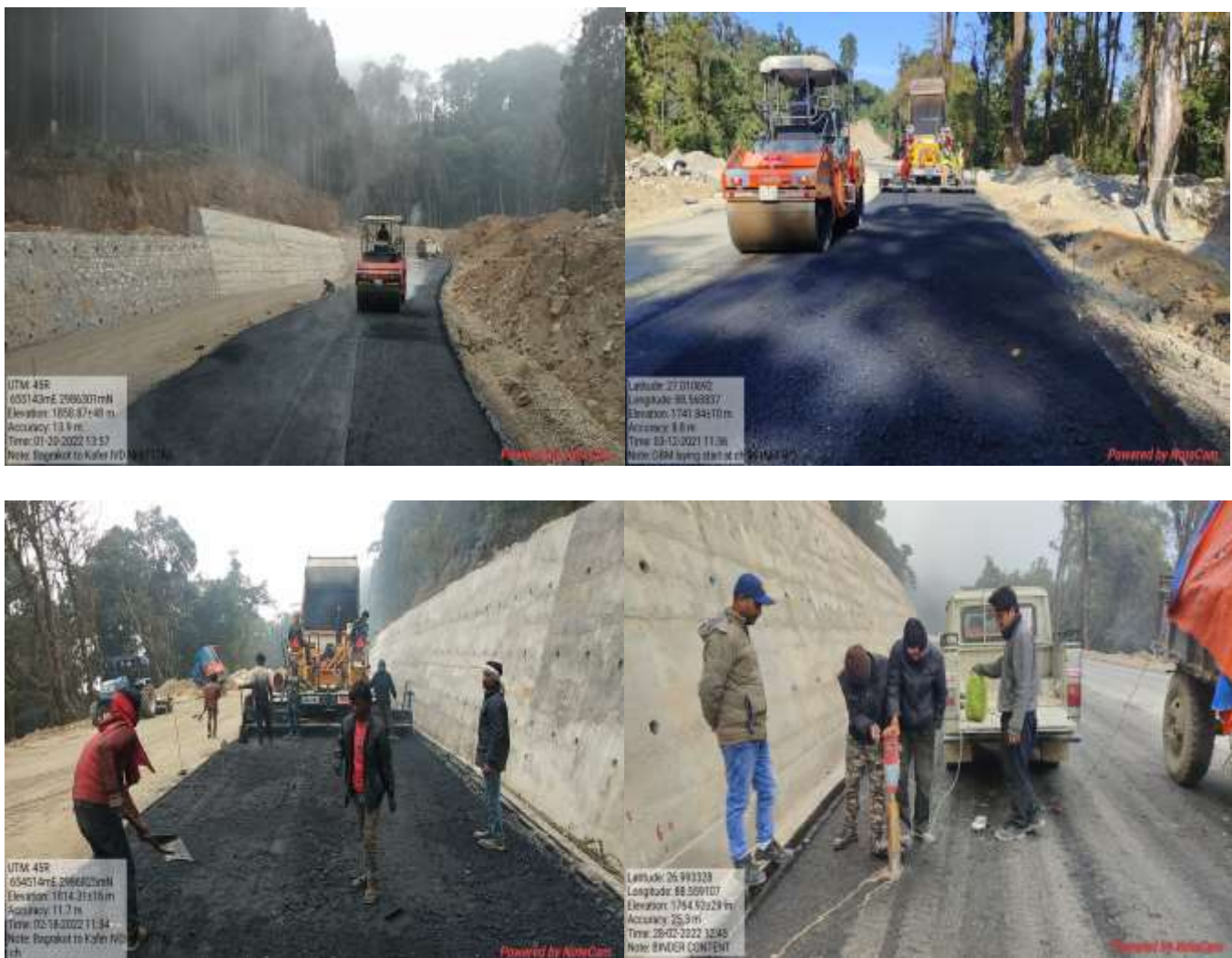
Photograph: 4.1: Laying of pavement layers i.e. DBM
