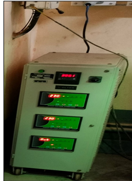
Fig. 3.2. Voltage Stabilizer
