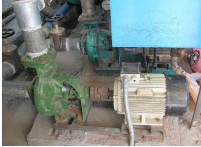
Fig 5.3 Pump used to recirculate the flow
