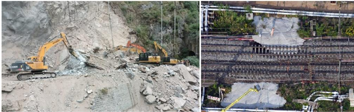
Figure 1.1 (a) Failure of an under-construction tunnel in Ramban district, J&K, May 2022 (b) Rastatt tunnel collapse, Germany, considered as of the most classic examples of tunnel failure. It consisted of twin track railway corridor between Germany and Switzerland. It was being constructed with the support of horizontal ground freezing through water-bearing sands and gravels. But failed with failure of the ground freezing regime and loss of integrity of the segmental lining, allowing ground loss under the rail tracks into the new tunnel bore beneath.
