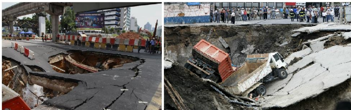
Figure 1.2 (a) Underground tunnel collapse causing a sinkhole in Kuala Lumpur, July 2014 (b) Sao Paulo tunnel failure due to “systemic failure” of design, construction and risk management, January 2007.
