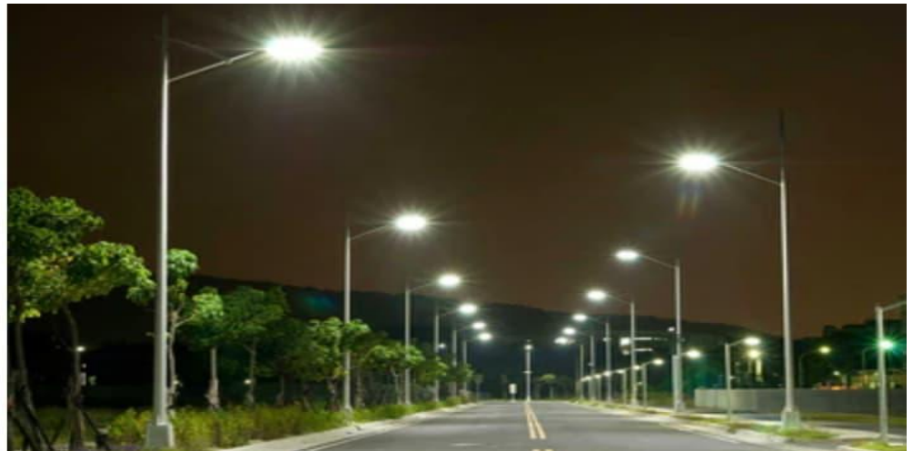
Fig 2.10. Staggered arrangement (two-sided arrangement offset)
