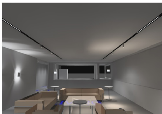
Figure 1.1: Track Lighting
