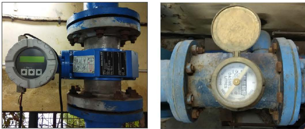
Fig. 3.5. Flow measuring instruments: (a) digital type and (b) analogue type.
