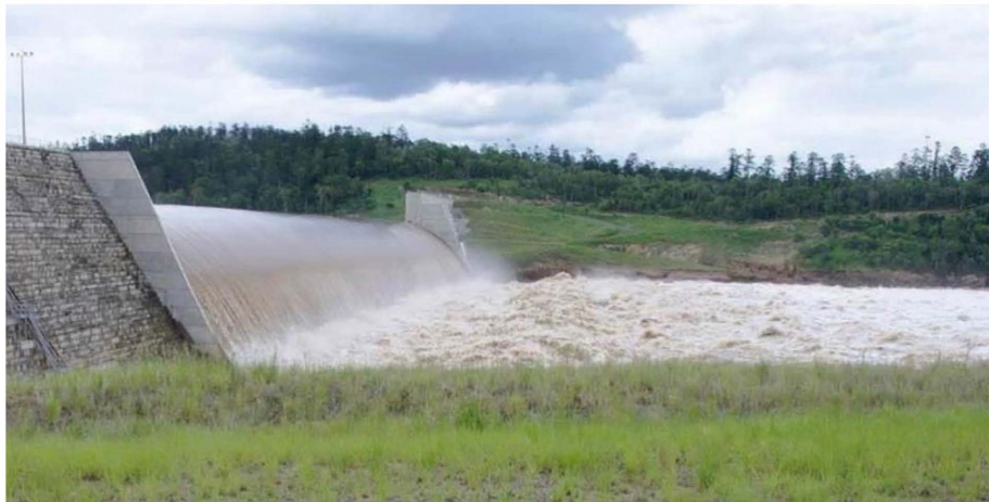
Fig. 1.7. Occurance of H-jump over the concrete stilling basin of Paradise Dam on the Burnett River, Bundaberg, Queensland, Australia (Bahmanpouri 2019).
