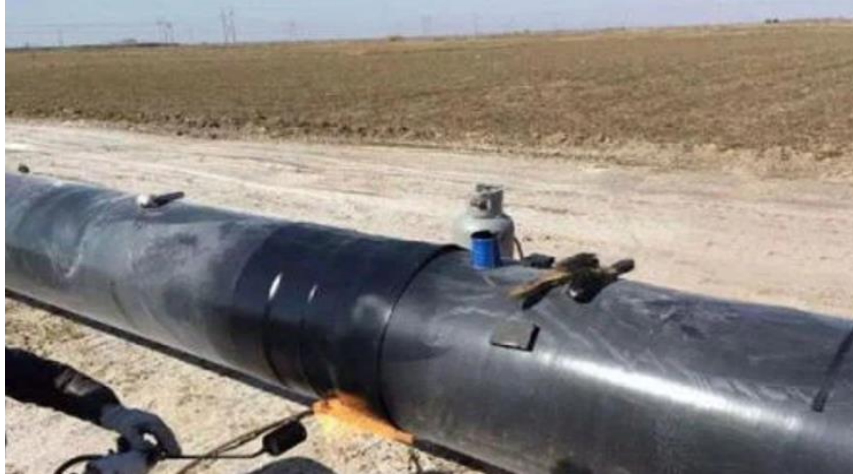
Figure 2.37: Application of PE-based HSS wrap on a Pipeline Bend Joint
