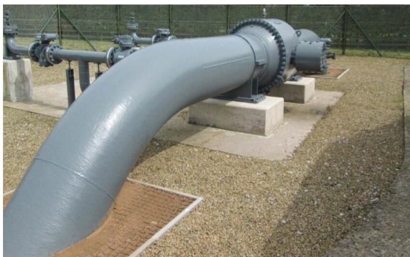
Figure 2.33: Solvent-Free Liquid-Applied Epoxy Coated Steel Pipeline
