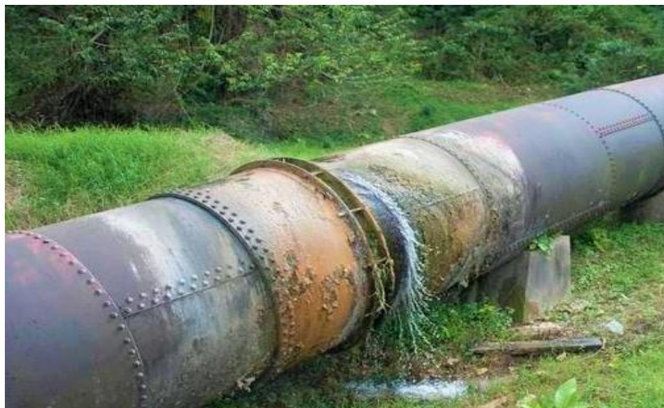
Fig.2.2: Water pipeline Corrosion
