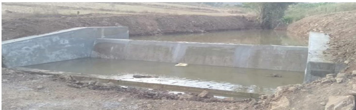
Pic -5.3: Check dam has constructed on irrigation canal in study area
