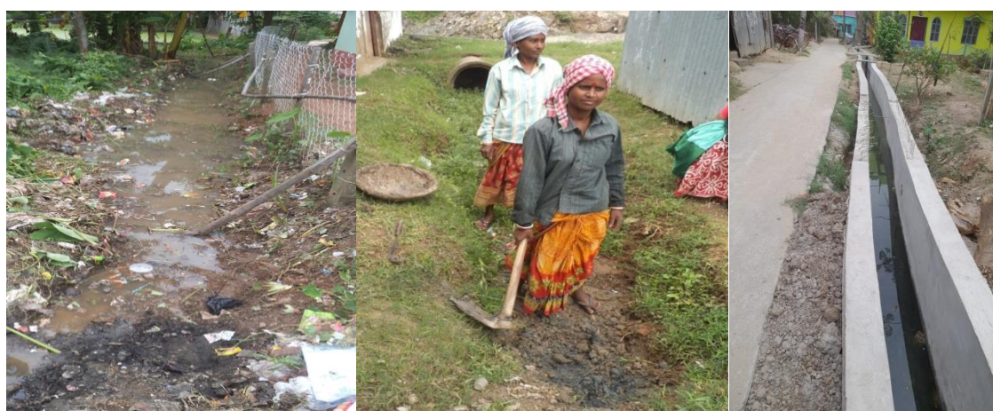
Pic - 5.6: (i) Improving the depth of drainage by removing garbage, (ii) Desilting of drainage, (iii) Concrete drain with strengthening of embankment in study area
