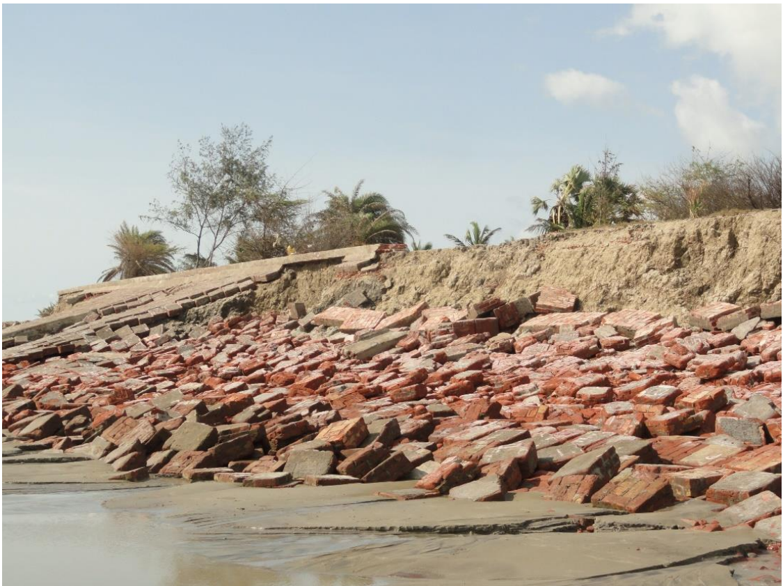
Photo 5. Breaching of embankments in the western part of the IBD
