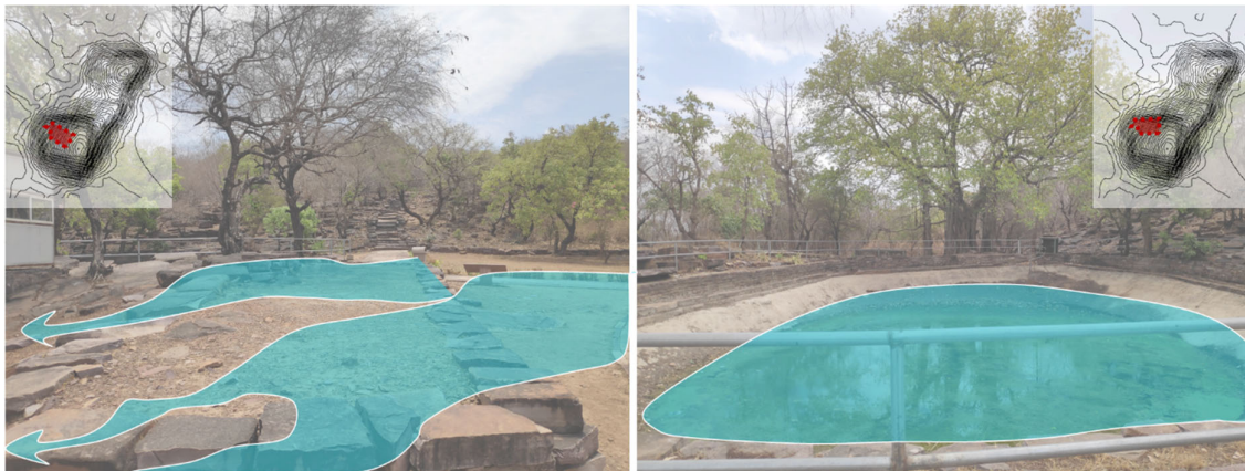
Figure 5-15: Terraced flow of surface runoff to manmade rainwater collection tanks (Source: Site documentation by author)
