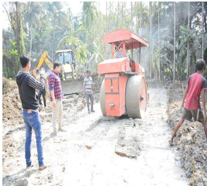
Fig. 6.15: Preparation of subgrade
