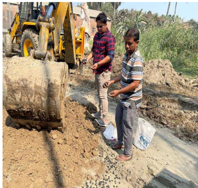
Fig. 6.14: Scrap tyre mixing with subgrade soil
