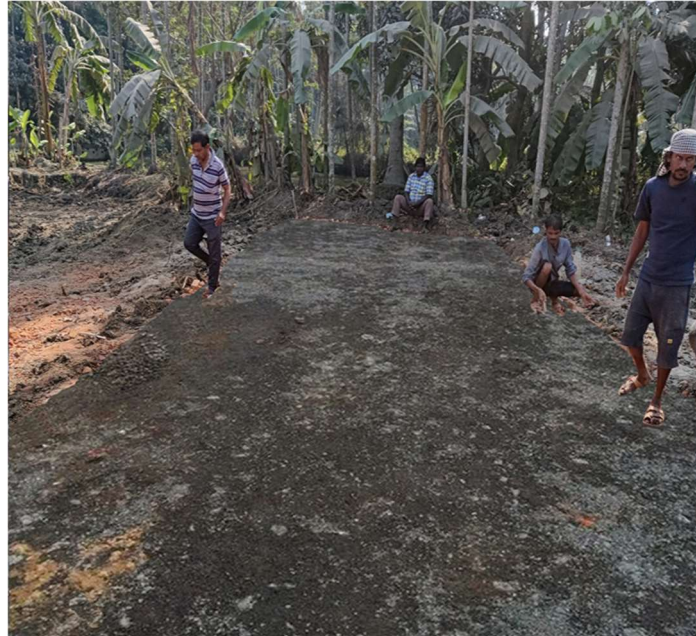
Fig. 6.16: Preparation of subbase layer
