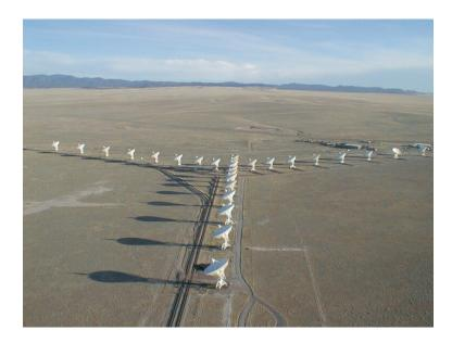
Figure 3.1: An aerial view of the Very Large Array and its 'Y-shaped' arrangement (Courtesy: NRAO).
