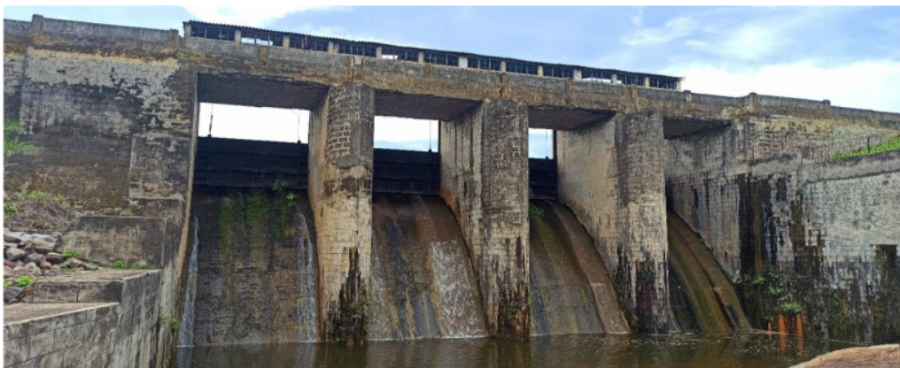
Figure 3.5g Spillway gates of Shali reservoir
