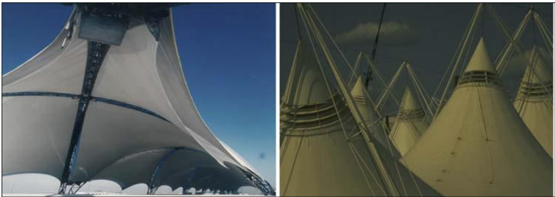
Plate 8.5.2: Double PVC covering and single covering with heat dissipation on the top and surface cooling via irrigation
