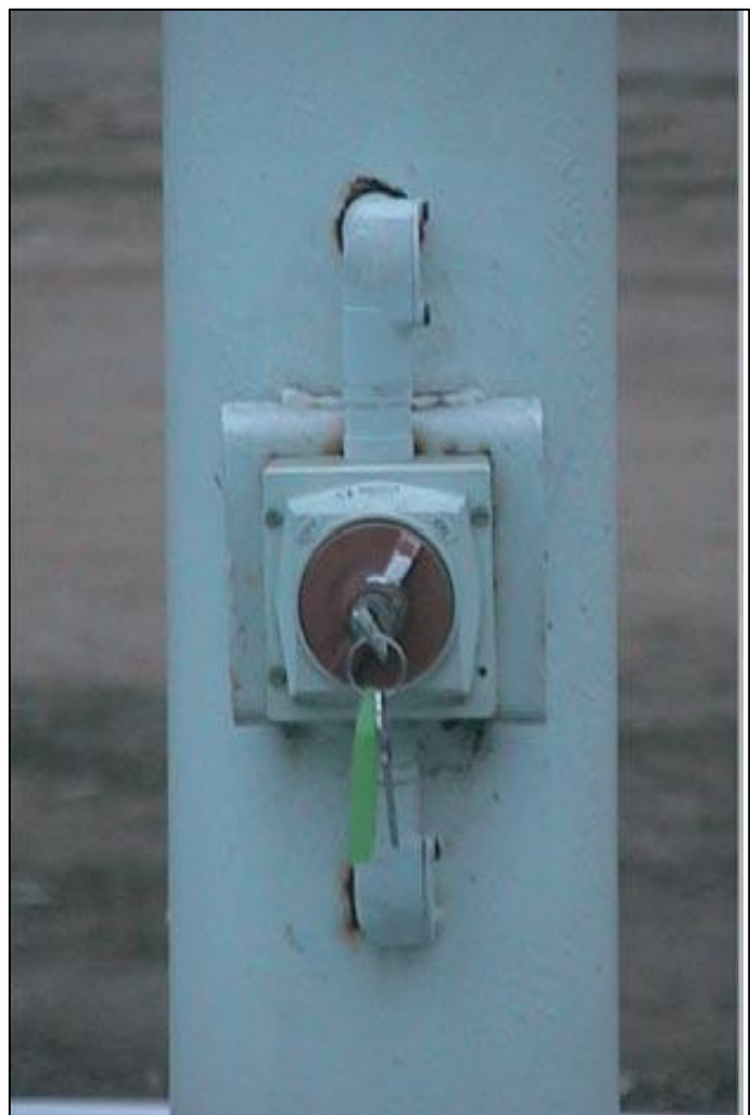
Fig-5.4: The pole is permanently wired from the club switchboard. A key switch at the base of the pole provides lighting control of a playing surface
