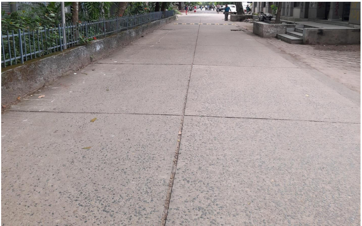
Figure 3(l): Concrete cement road surface used in this experiment
