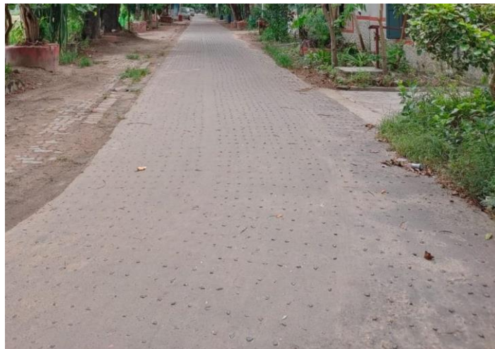
Figure 3(c): Asphalt Mastic Road surface used in test
