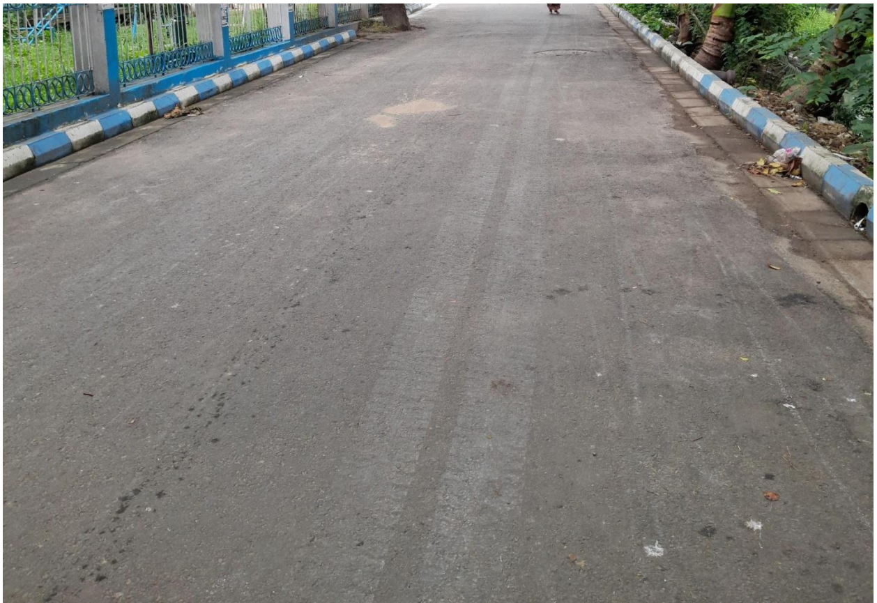
Figure 3(f): Bituminous asphalt road surface used in this experiment
