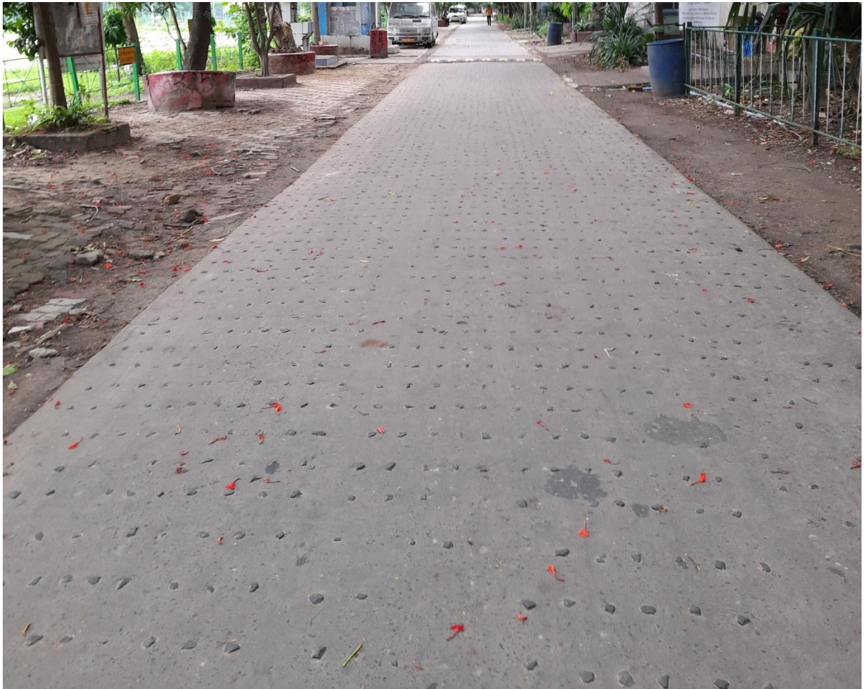
Figure 3(b): Asphalt Mastic Road surface used in the test
