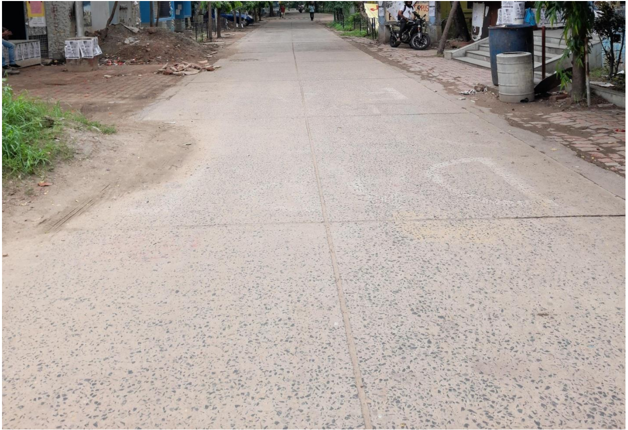
Figure 3(k): Concrete Road surface used in the experiment
