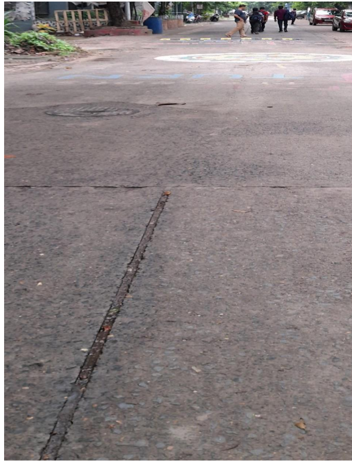
Figure 3(i): Concrete Road surface used in experiment
