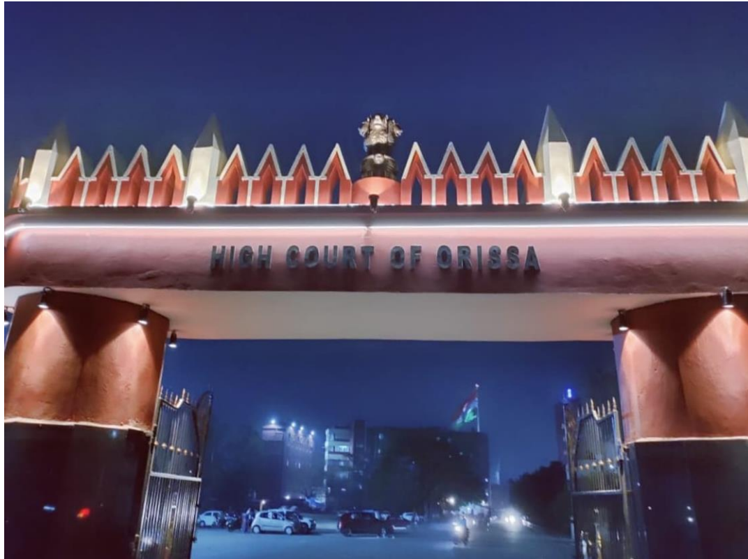
Fig 7.15: Picture taken after lighting installation (Front View)
