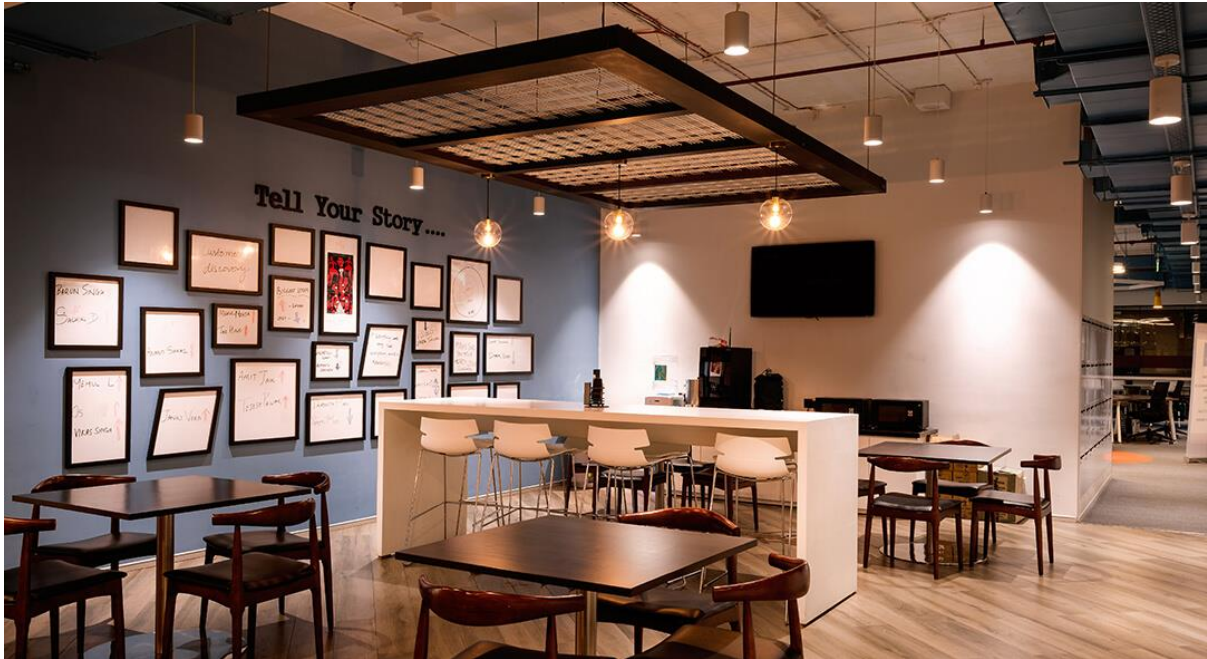
Fig 1.1: Indoor Decorative Lighting Design with suspended luminaires [1]
