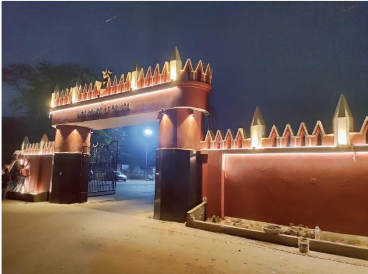
Fig 7.16: Picture taken after lighting installation (Side View)
