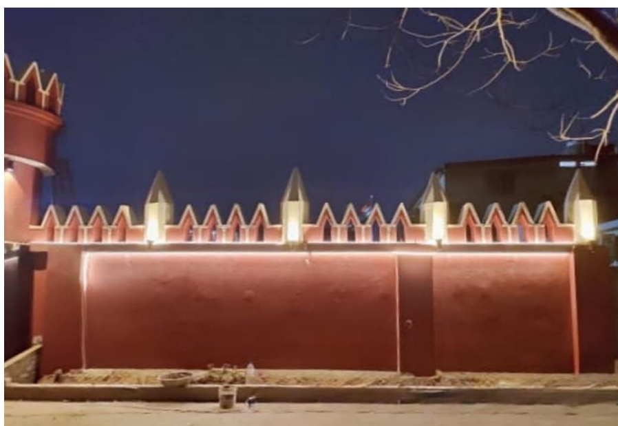
Fig 7.16: Picture taken after lighting installation (Right wall)
