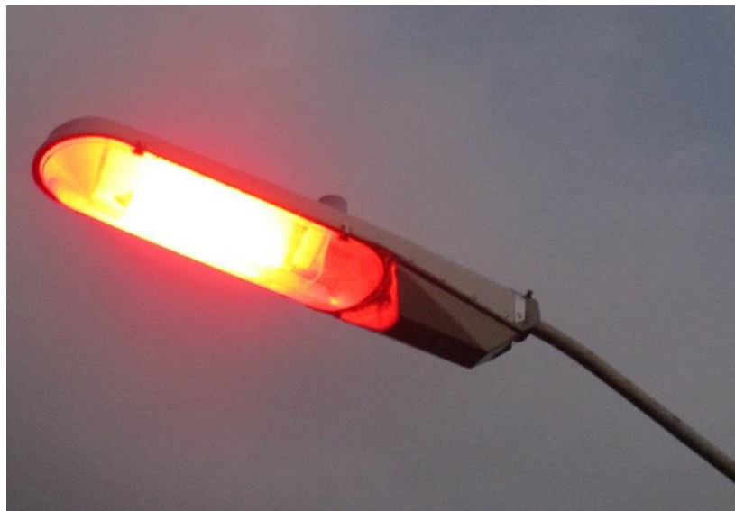
Fig 3.6 : LPS lamp luminaire mounted on street light pole.
