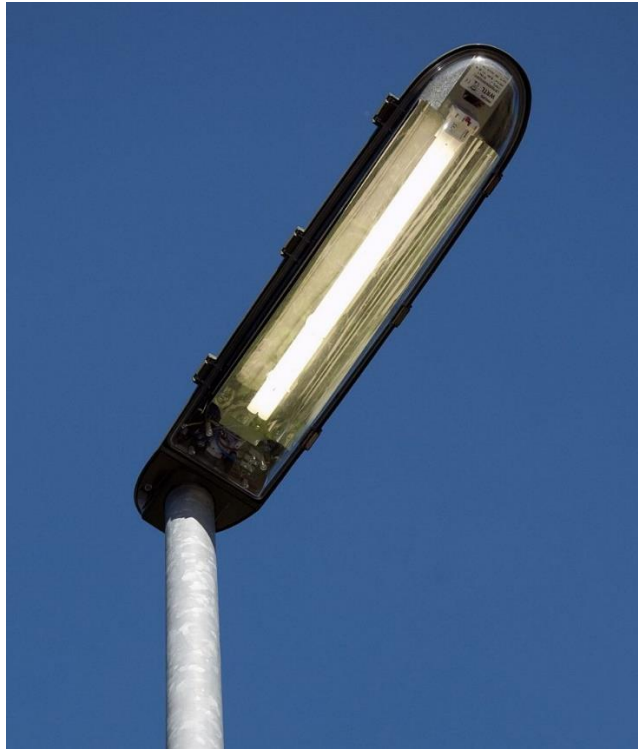
Fig 3.11 : Fluorescent lamp luminaire mounted on street light pole.
