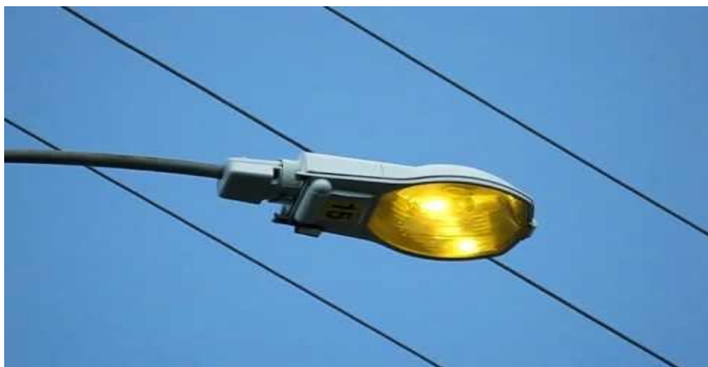
Fig 3.8 : HPS lamp luminaire mounted on street light pole.
