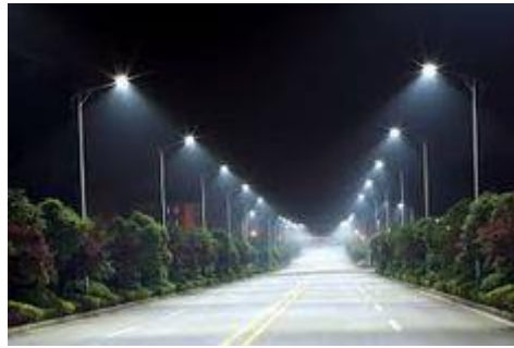
Fig 1.1 Example of Street lighting
