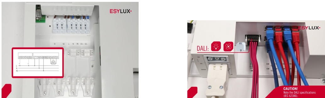
Figure 43: Connection of Smart-Driver
