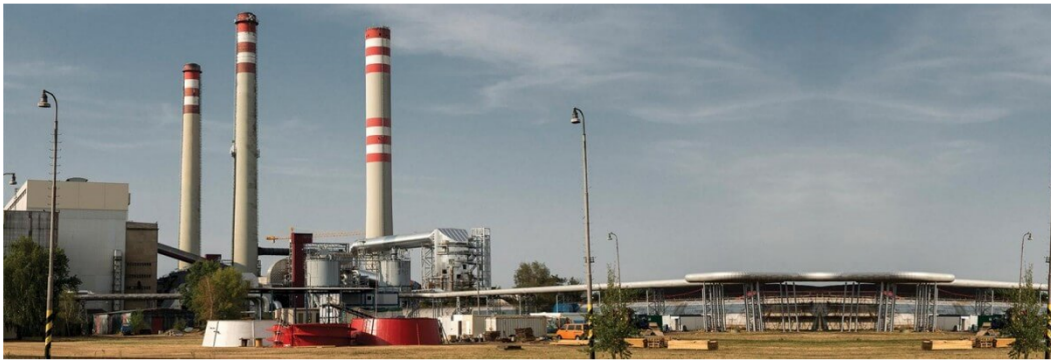
Figure 4.11: Wet stack (Chimney)
