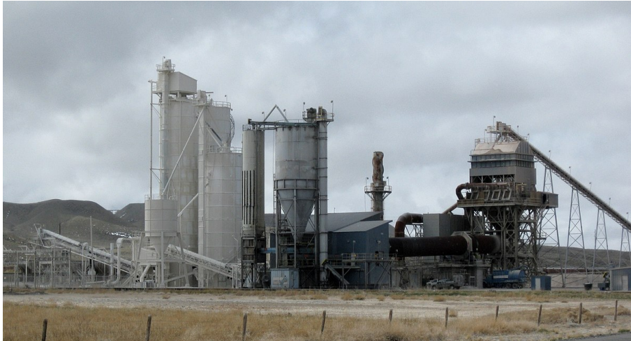
Figure 4.7: Limestone Terminal Point
