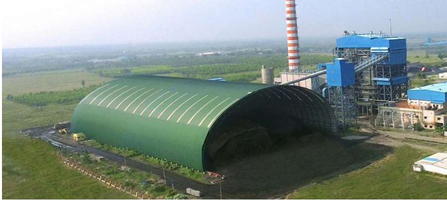
Figure 4.3: Gypsum Storage Shed
