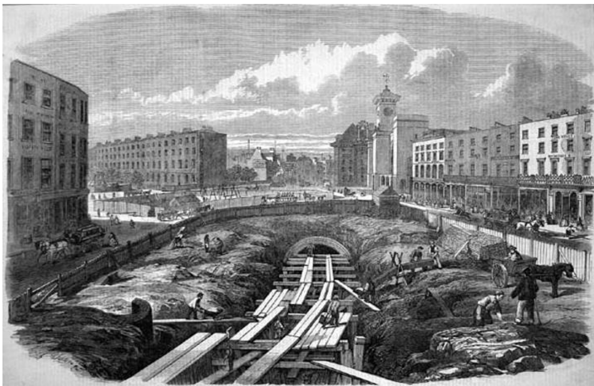
Fig 1.1 Initial construction stages of London's Metropolitan Railway in 1861
