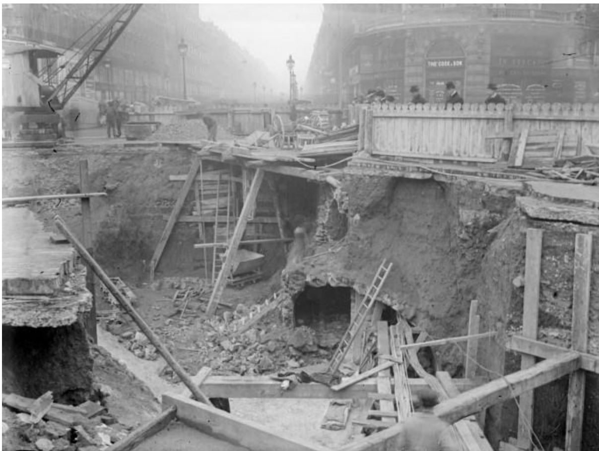
Fig 1.3 Paris Métro under construction around 1900
