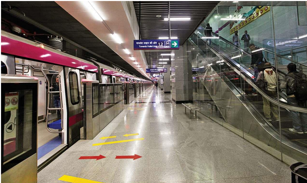
Fig 5.33 Real Time Image of Underground Metro Platform
