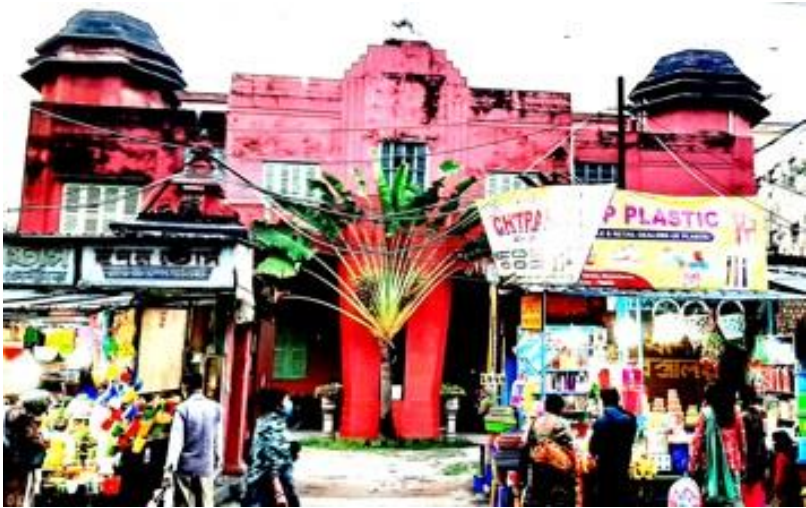
Picture 34: Well-maintained old structures, zone I. Source: Author
