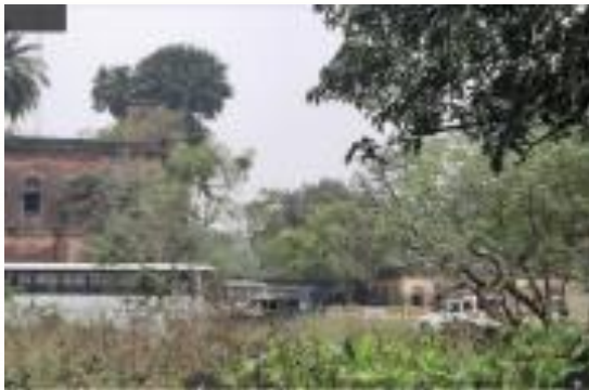
M5 - Lalkuthi Fire Station (Old Building)
