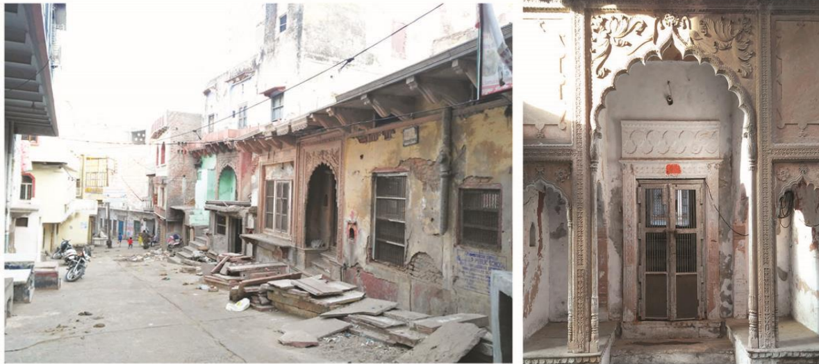
Figure 15 Religious assets in dilapidated conditions
