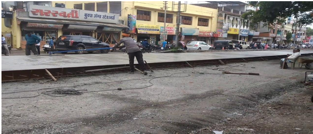
Fig. 1.5: Dry Lean Concrete Base for Rigid Pavement
