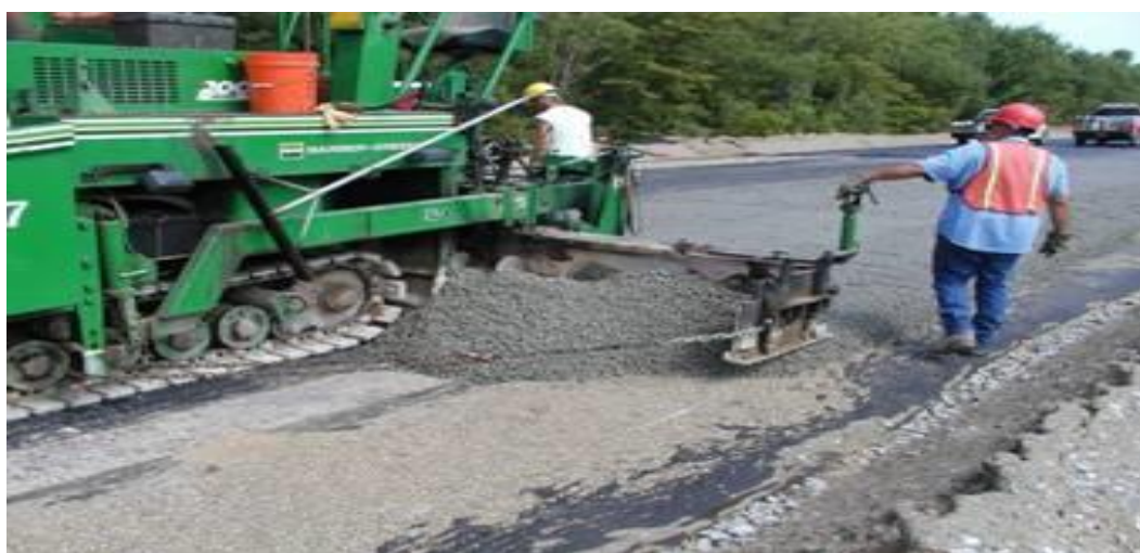
Fig. 1.6: Construction of base for road pavement by Dry Lean Concrete.
