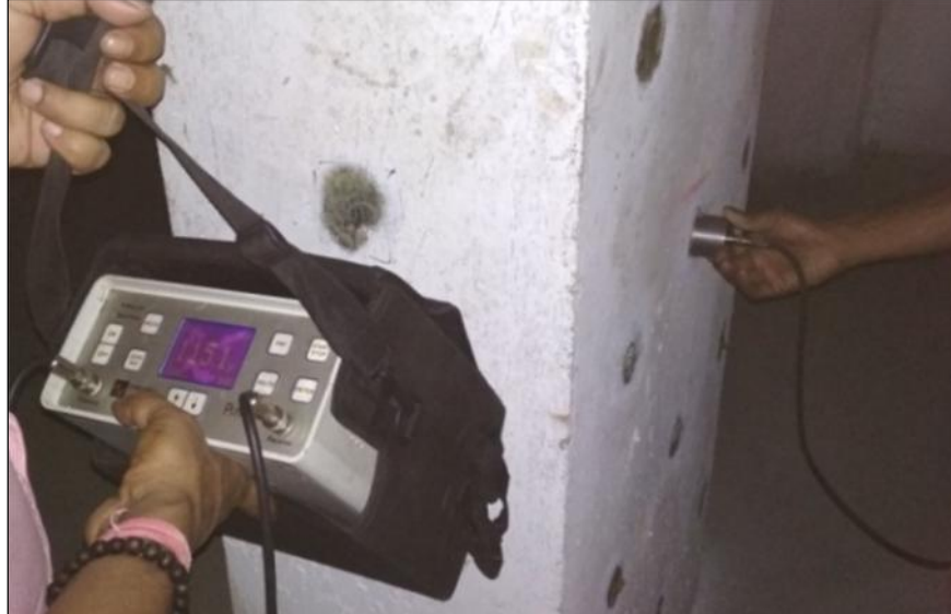
Fig-4.3: Ultrasonic Pulse Velocity assess the Quality of Concrete
