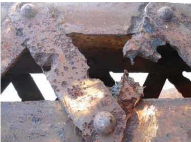
Fig 5: Pitting Corrosion
