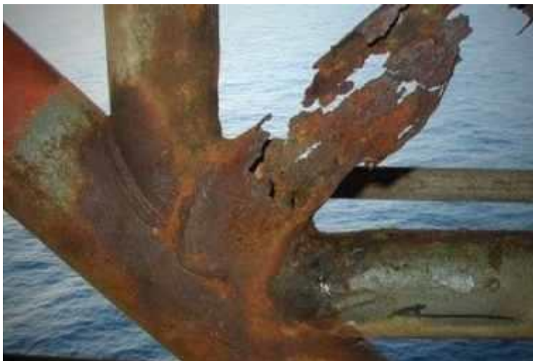
Fig 9 corrosion fatigue
