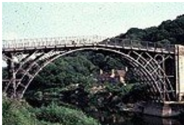
Coalbrookdale bridge, England First Cast-Iron Bridge
