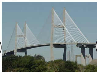
Prestressed concrete, Cable stayed bridge
