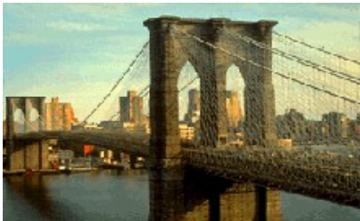
Suspension Bridge Steel suspenders
