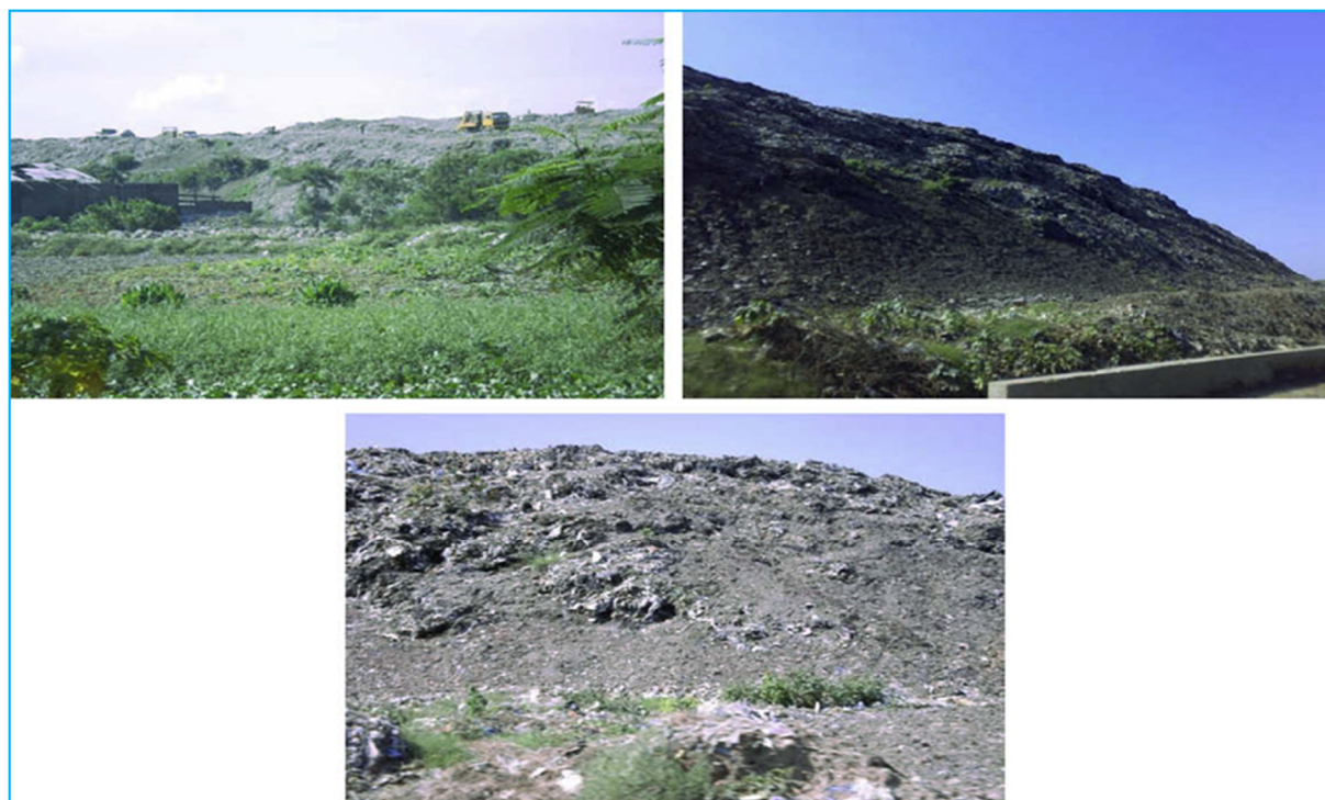
Fig. 24: Dhapa Dumping Site, waste piles are 17 m high from ground level. ( Hazra et al., 2009)
