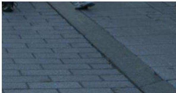
Figure 82 curb stone to define diverse lanes
