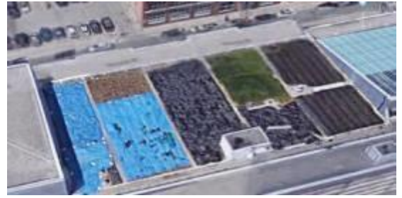
Figure 89 Vari green roof
