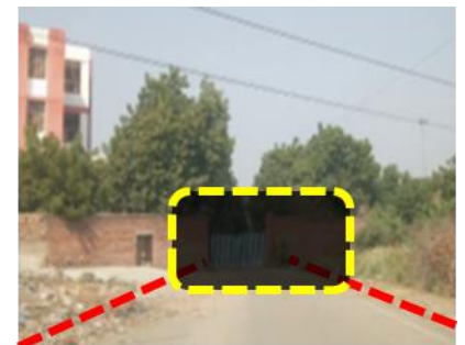
Figure 130 Blockage of road
