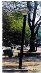
Street lights for walkways
