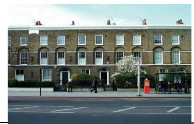
Figure 32 - Images of Architectural features study
