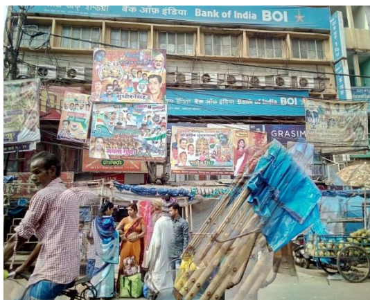
Elevation Of Building Obstructed By Different Wire
