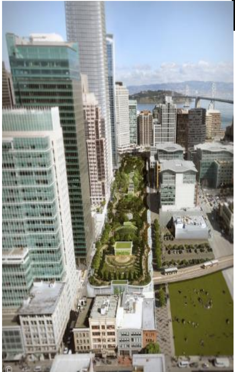
Fig 22 :View of transbay terminal
