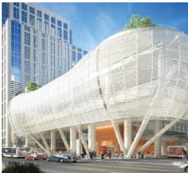
Fig 21 :The terminal as seen from Beale Street
