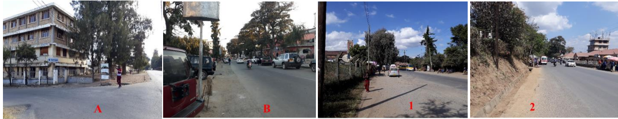
The pictures show the existing road condition refer figures above
