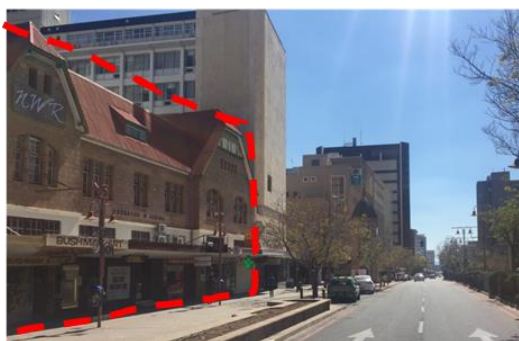
Fig. 2.20 Historical building at CBD Source: Google Street view, 2019
