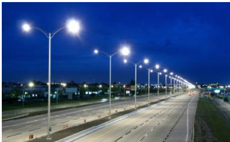
Fig 1.1: Road lighting luminaires showing visual guidance of the path
