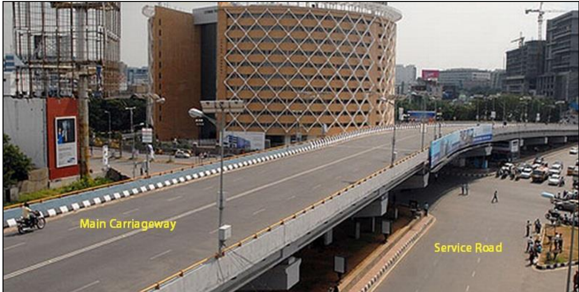
Fig 2.3B: Main Carriageway and Service Road
