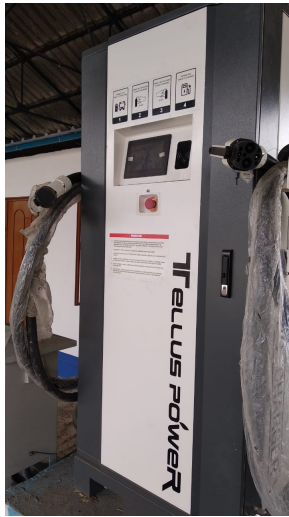
Figure 2.2: first charger installation in lake depot
