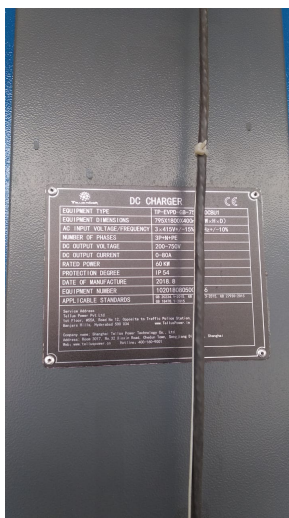
Figure 2.4: Rating template of the DC charger
