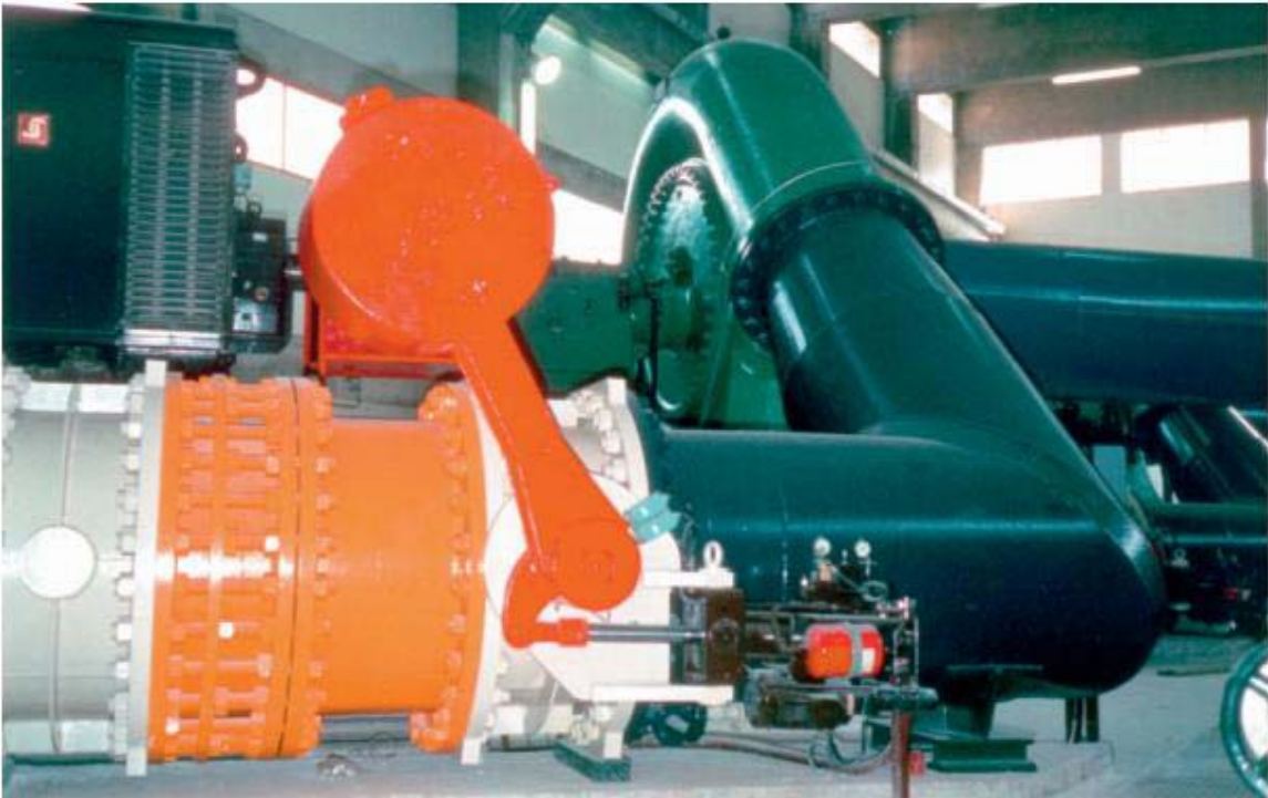
Fig 2.9: Swing check valve equipped with a hydraulic actuator and counterweight
