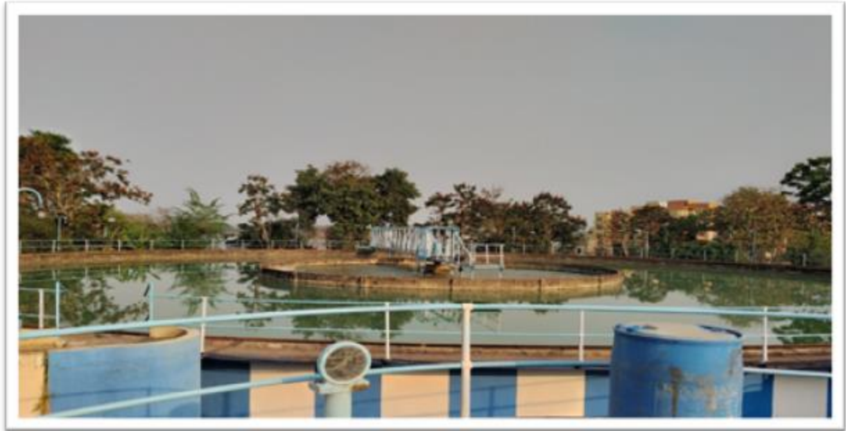
Figure 3.3 Clariflocculator
