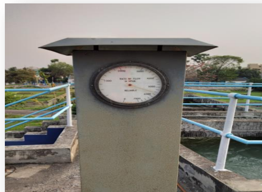
Figure 3.2 Flow Meter
