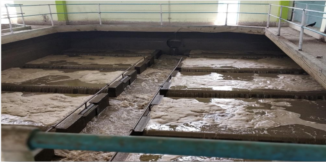
Figure 3.5 Backwashing of Filter Bed
