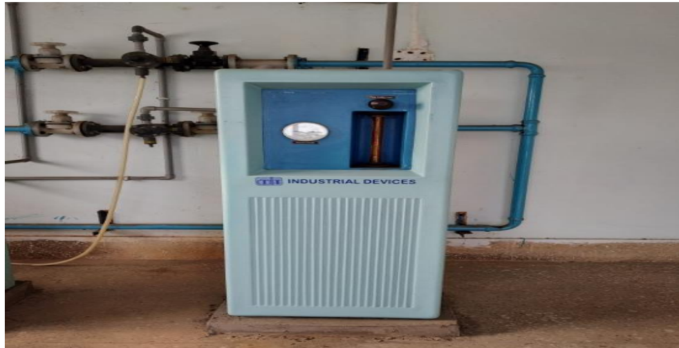
Figure 3.8 Chlorinator
