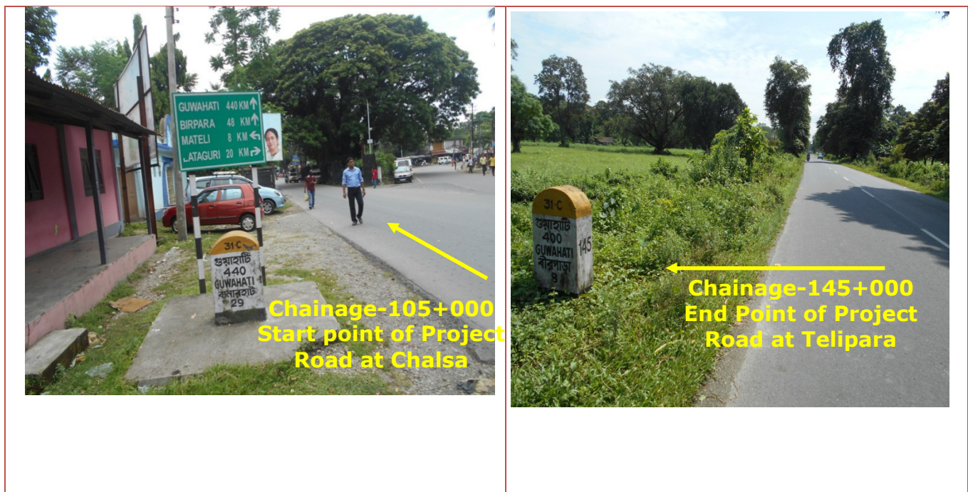
Photograph 1.1: Start and end point of the project corridor
