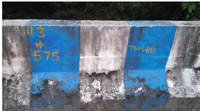
Photograph 5.1: Fixing of chainage on culvert
