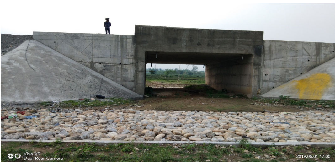
Photograph 3.3: Some photograph of ongoing work at study Area
