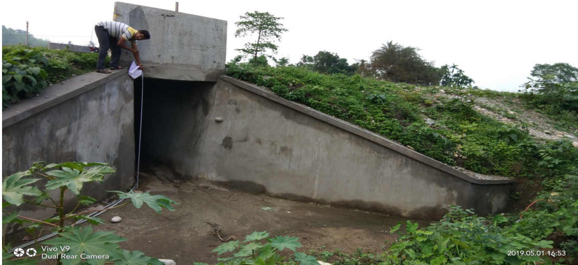
Photograph 4.9: Taking measurement of the existing culvert
