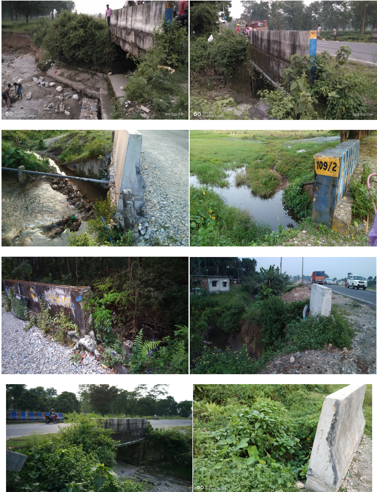
Photograph 3.2- Existing culvert & Bridge at study Area
