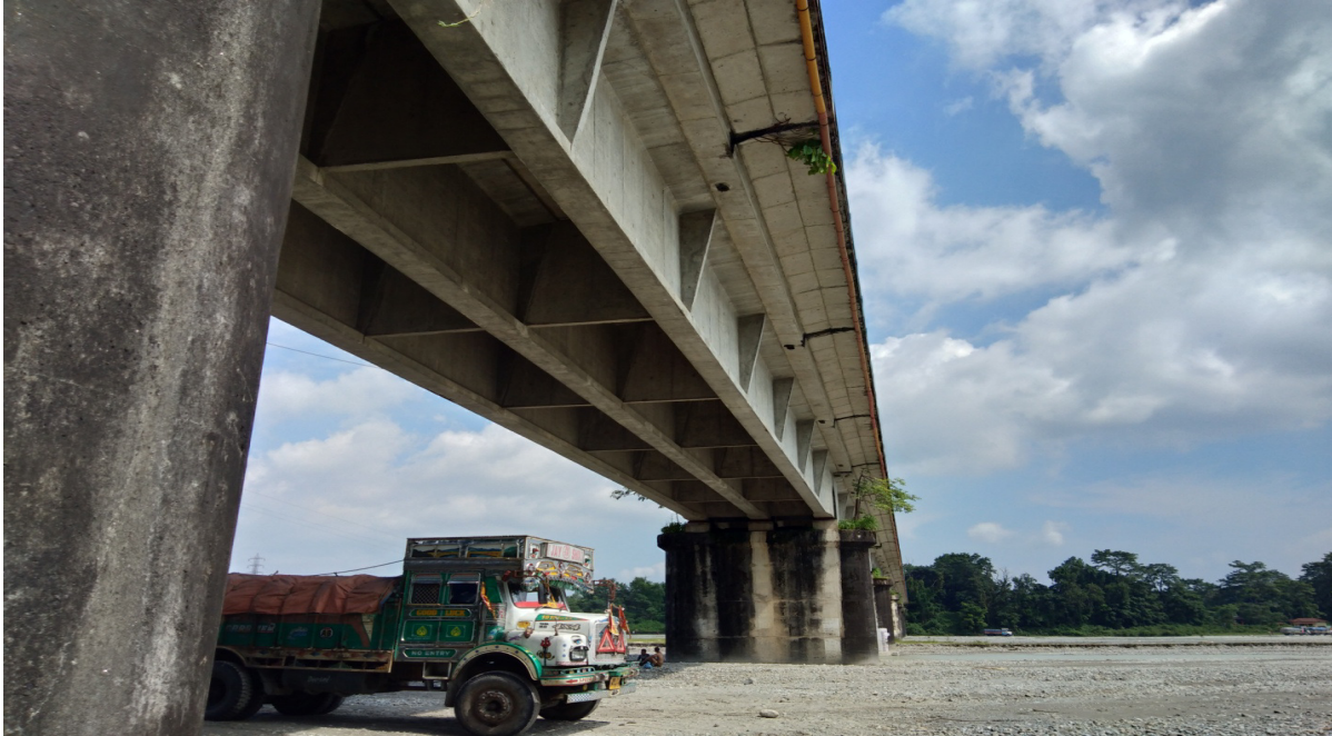
Photograph 4.8: Image of major Bridge condition from bed
