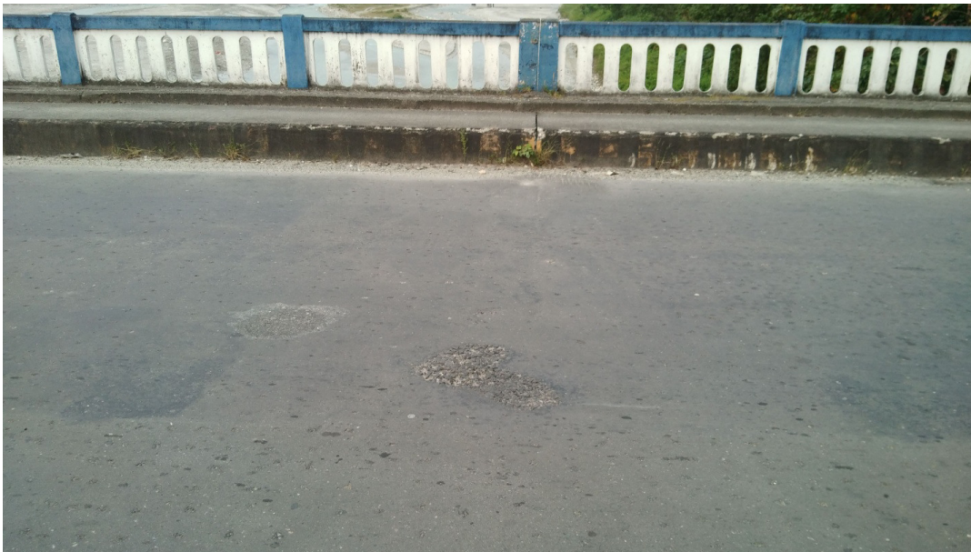
Photograph 4.5: Patching work on project corridor
