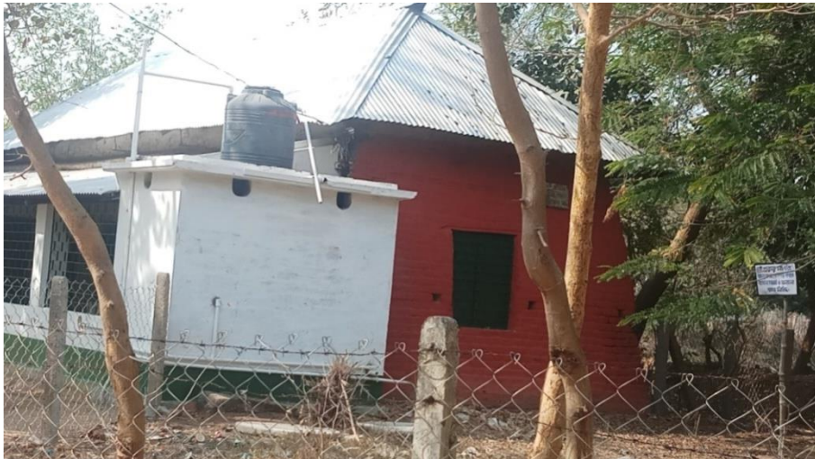
Mirzapur WTP situated at a this remote village
