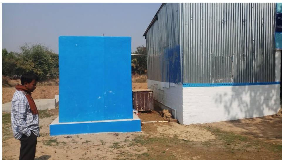
Various unit of Treatment Plant
