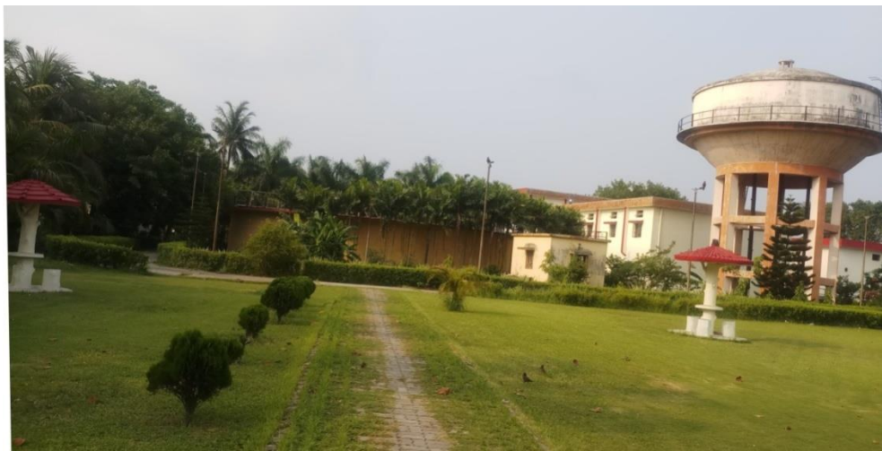
Overhead Storage Tank & Storage After Purification Before Distribution
