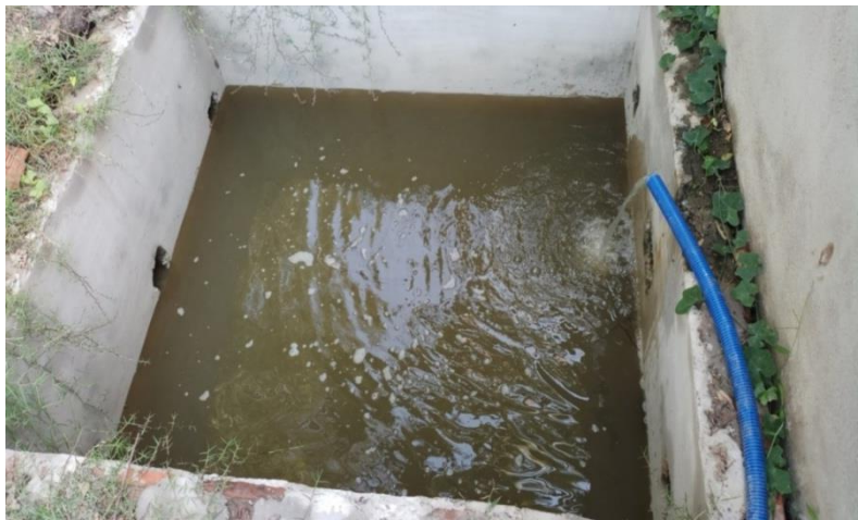
Underground recharge process by wastage water
