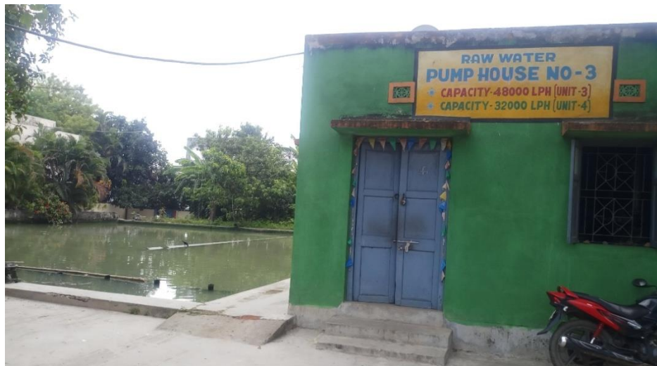
Raw Water/Pump House
