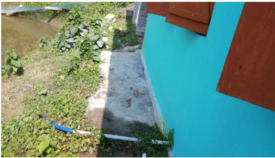
Pond for supply raw water
