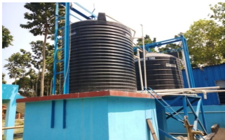
Raw Water Collection Reservoir
