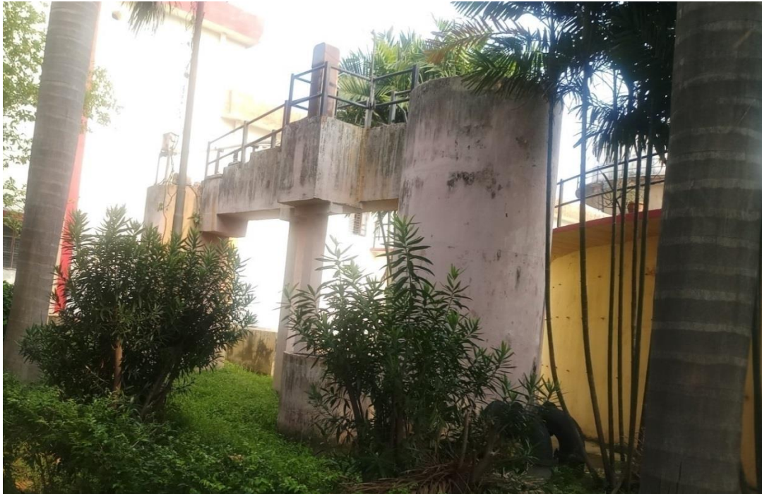
Intake Water Connected With Solution Of Alum & Chlorine.
