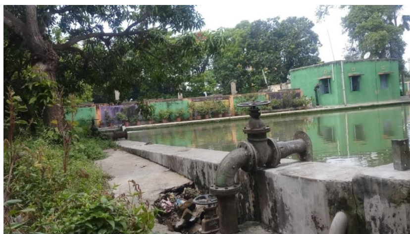
Intake of raw water Figure-5.5.4
