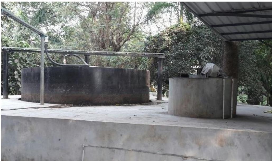
Mesophilic digester, floating drum gas holders, and feeding tank
