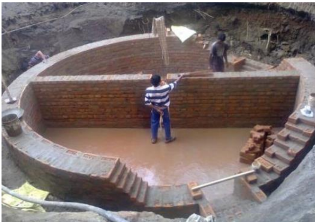
Mesophilic Digester during construction
